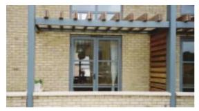
Although the doors and windows on this development are of an appropriate standard, security is compromised by design features that make access to upper levels easier.
