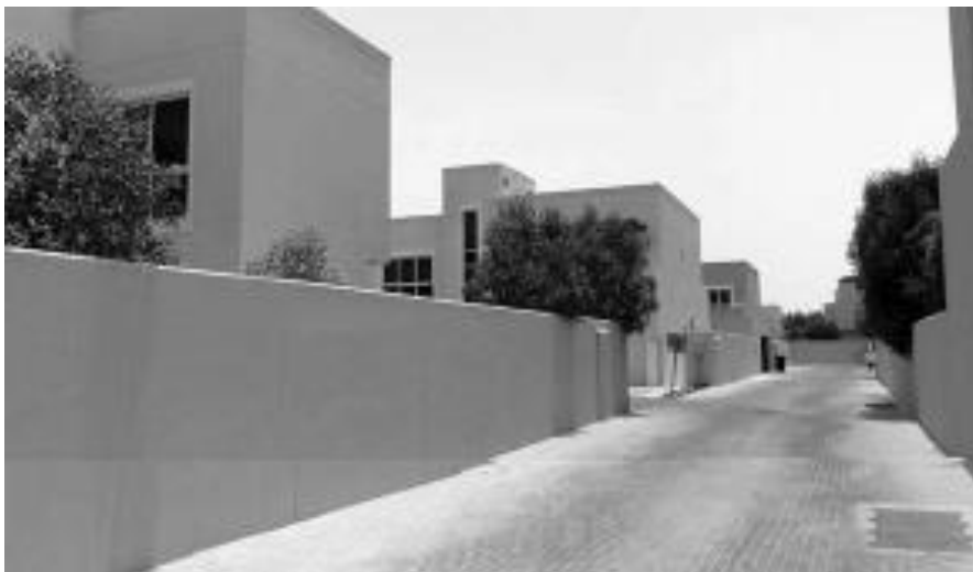
Figure 3 Boundary walls restrict levels of surveillance.
